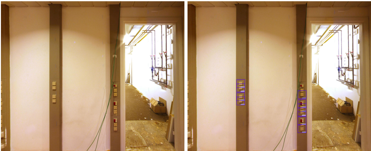
Figure 10: The ElecDetect module performs the detection of sockets and switches (right) on orthophotos generated by the OrthoGen module (left).
